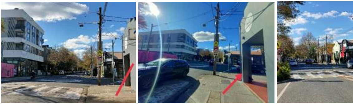
3 storey Structure at corner of Mitchell Road and Maddox Street Alexandria at 1pm on 25th June 2025
