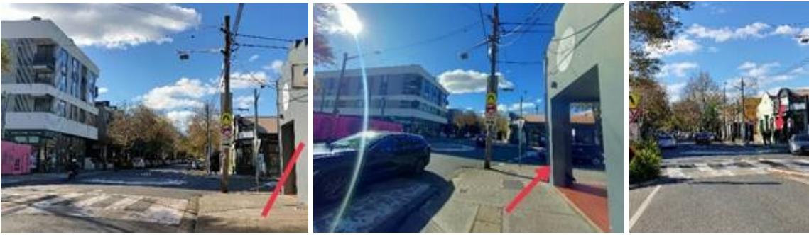
3 storey Structure at corner of Mitchell Road and Maddox Street Alexandria at 1pm on 25th June 2025
